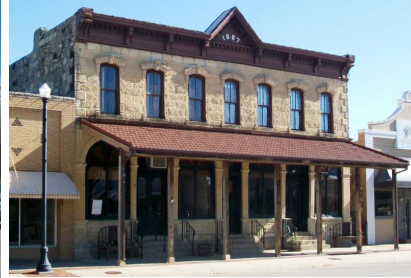
Commercial Building. 126 N Main Street. West Elevation. Looking SE. Photo by William E. Fischer, Jr., 11/11/2011
